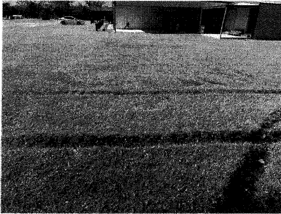
PHOTOGRAPH DESCRIPTION: Ruts in Becky's Catering property west of entrance drive to EWST #1 site. Standing west of entrance drive looking west in line with the front of building.
